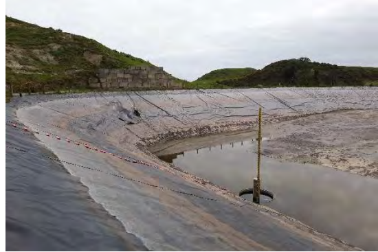
Tomo showing after Bottom Drain down
