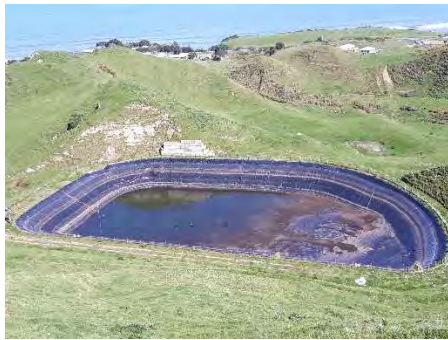
Bottom storage dam (drained out)
